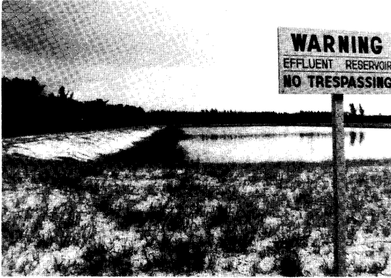
Sewage treatment effluent reservoir, or holding pond.
