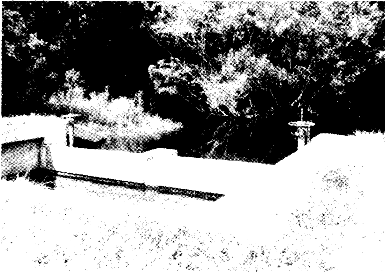
Water management weir for maintaining water levels in the Sanibel River.
